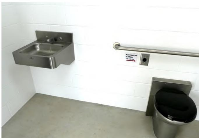
*Flush toilet and sink for handwashing are standard with flush-vault units. A urinal is also included.*
