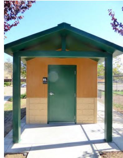
*Flush-vault unit installed by City of Lathrop at new dog park went eight months before it needed pumping out*
