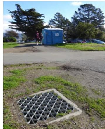
*Existing storm drain box near restroom site is three feet deep and poses no exposure hazard*
